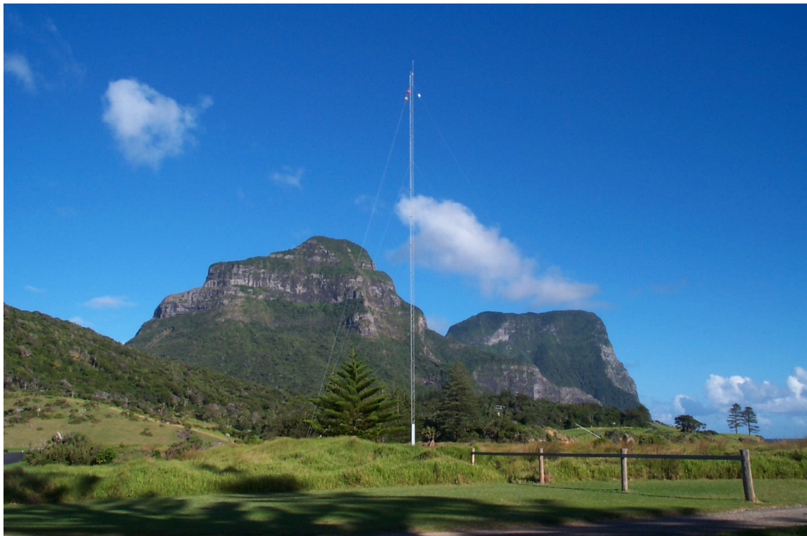
Figure 16 40m guyed lattice mast at the SEDA (NSW) monitoring site at Lord Howe Island
