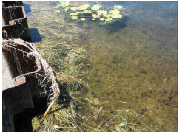
Figure 3-1 Sediment and Algae at Giru Weir
